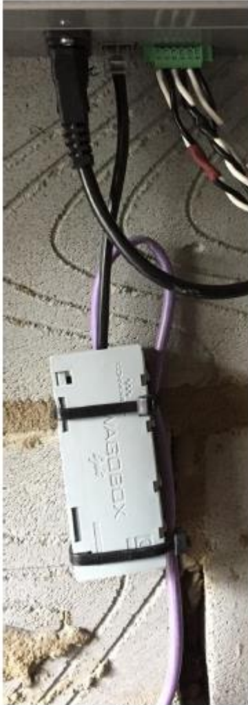
Figure 4 - Connecting the serial cable to the RJ45 socket on the hub
